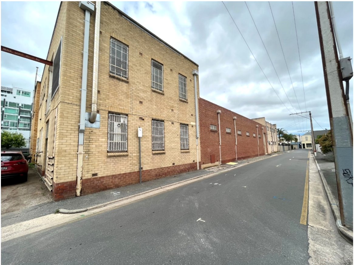
Photo 3.6 – adjacent Telstra Exchange site at 132-134 Ward Street looking south west
